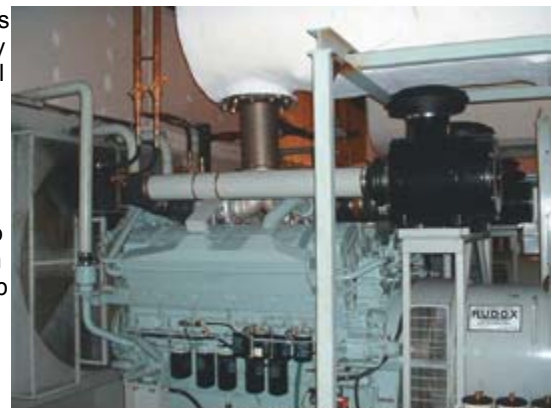
PHOTO: BROOKLYN UTILITY MANAGEMENT
