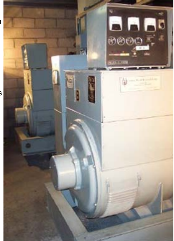
PHOTO: BROOKLYN UTILITY MANAGEMENT
