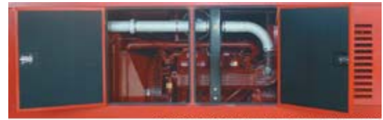
PHOTO: BROOKLYN UTILITY MANAGEMENT
