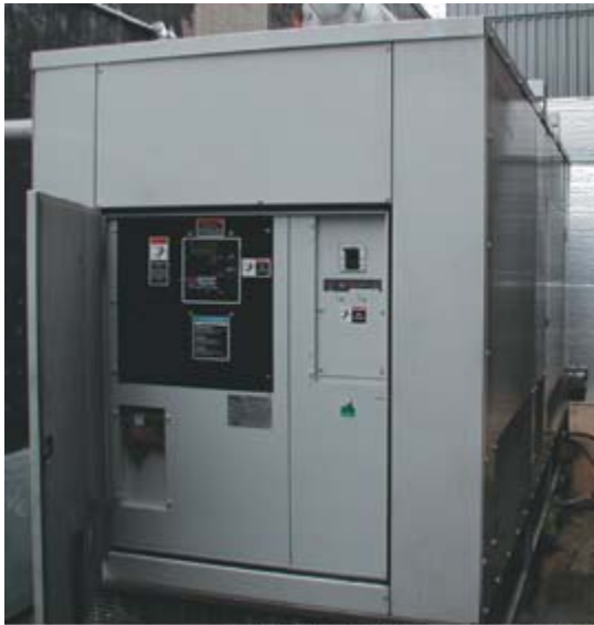
PHOTO: BROOKLYN UTILITY MANAGEMENT
