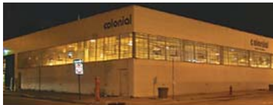
PHOTO: BROOKLYN UTILITY MANAGEMENT
