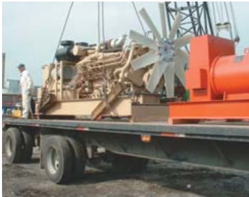
PHOTO: BROOKLYN UTILITY MANAGEMENT
