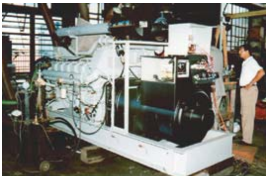
PHOTO: BROOKLYN UTILITY MANAGEMENT
